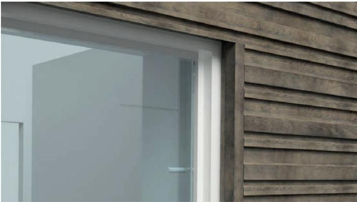
When using brads to fix Cladding and reveal boards around window/door openings, we would recommend the use of a clear polymer adhesive/sealant to help secure the products in place.
