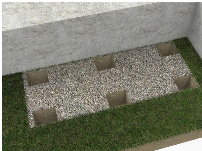
Holes for post supports dug as required. Min 400mm deep.
