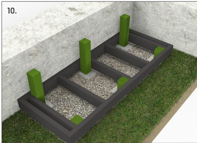
**h.** The 2nd step is now positioned at the correct height, set level and attached to the posts or supports from the 1st step. 50x50mm or 125x50mm offcuts can be used as these intermediate supports.
