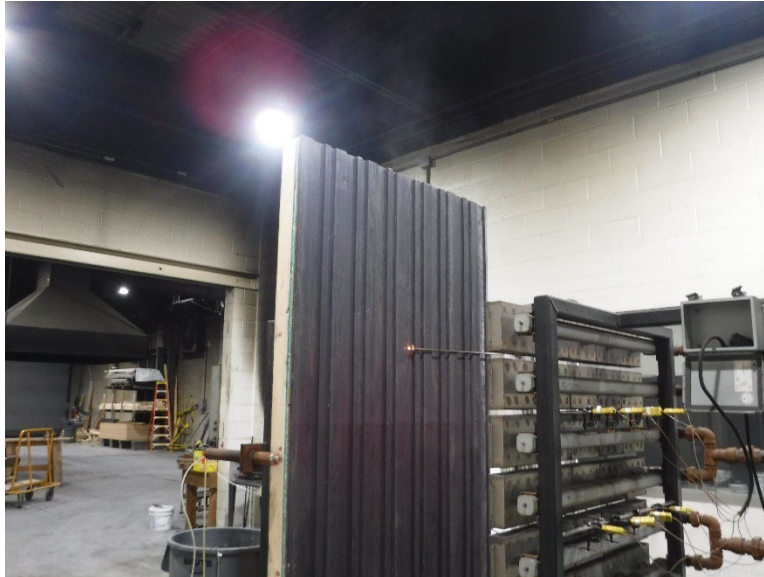
Photo No. 9 Smoke Emitting from Test Assembly
