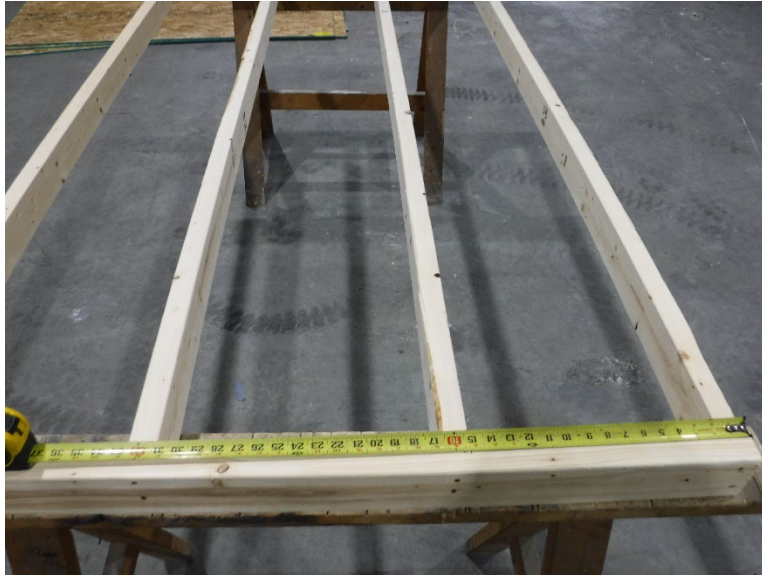
Photo No. 3 Wall Framing Spaced 16" on Center
