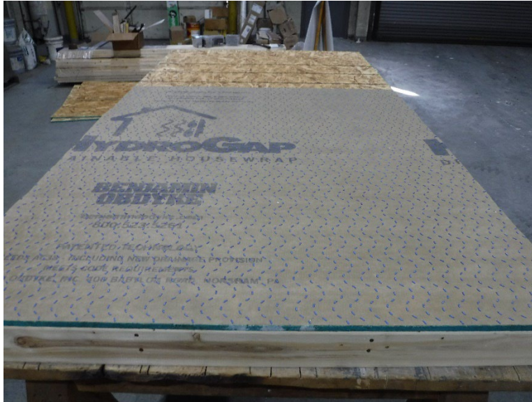
Photo No. 5 Addition of HydroGap®
