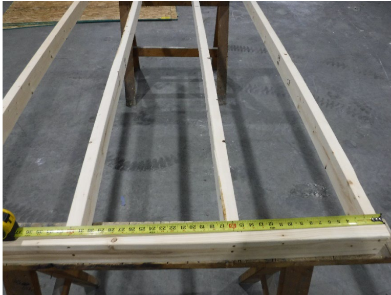
Photo No. 3 Wall Framing Spaced 16" on Center
