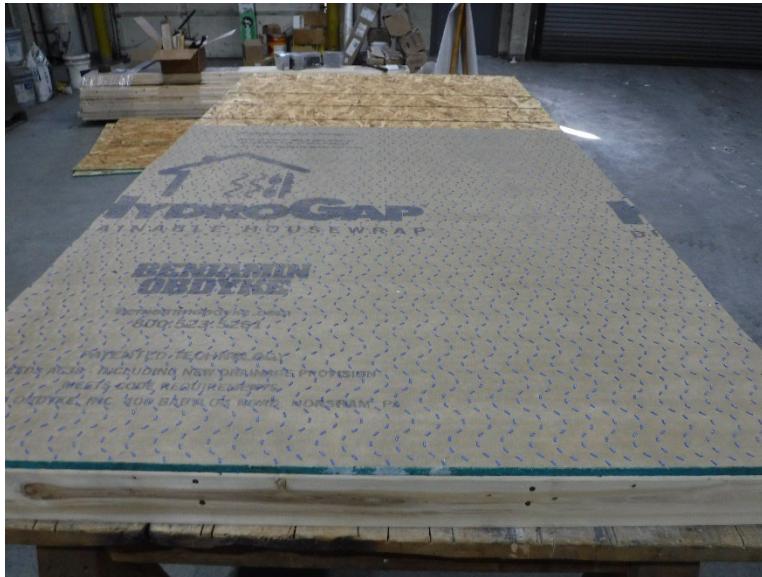
Photo No. 5 Addition of HydroGap®
